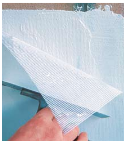
(5) Application of RIALTO FIBRELAST and leveling treatment with second coat of RIALTO RASELAST
