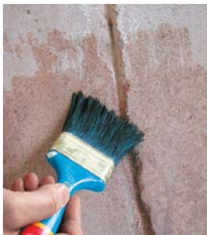
(2) Application of RIALTO PRIMER (interior walls) or RIALTO STABILIZER (exterior walls)
