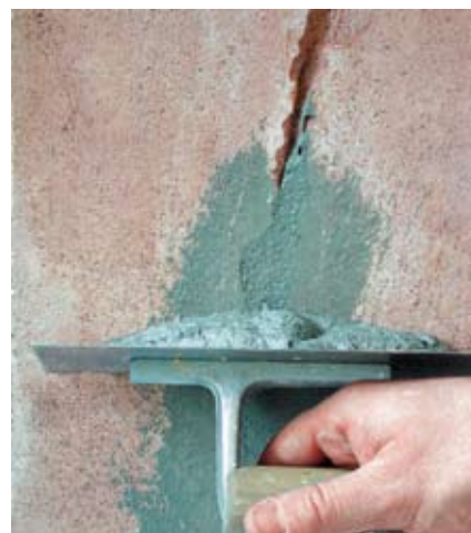
(3) Sealing the crack with RIALTO RASELAST mixed with cement
